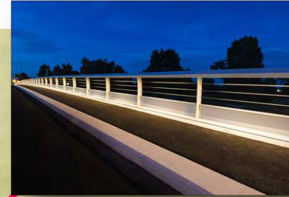
Linear Lighting at Bridge Rail
