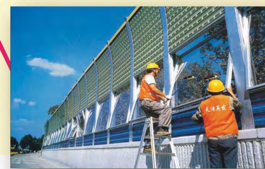
Transparent panels at bridge
