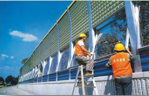
Transparent panels at bridge
