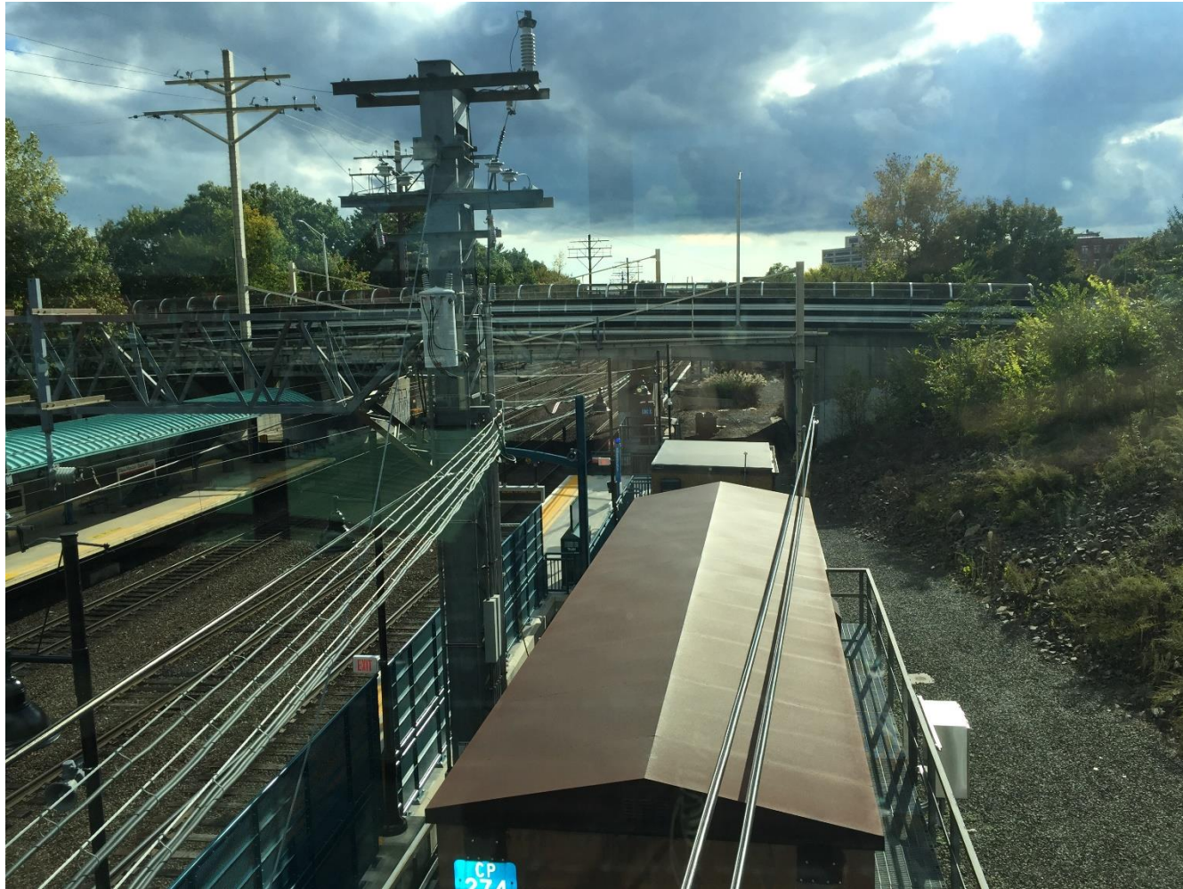
View of Bridge from Train Station Pedestrian bridge
