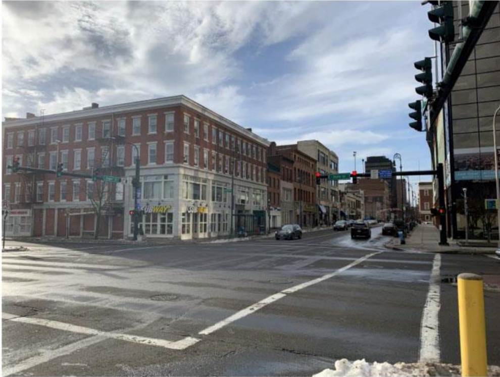
View from State Street Station. Corner of Chapel St. entering into Ninth Square where proposed archway will be installed
