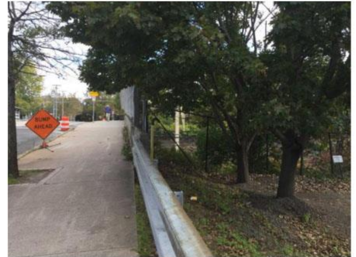
Natural overgrowth at the bridge endpoint on State St.
