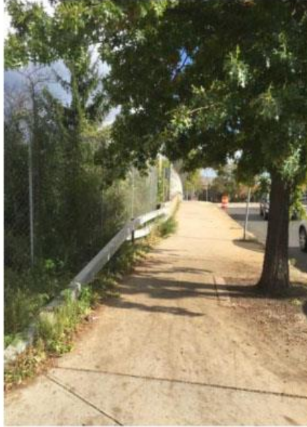
Natural overgrowth at the bridge endpoint on Union St.
